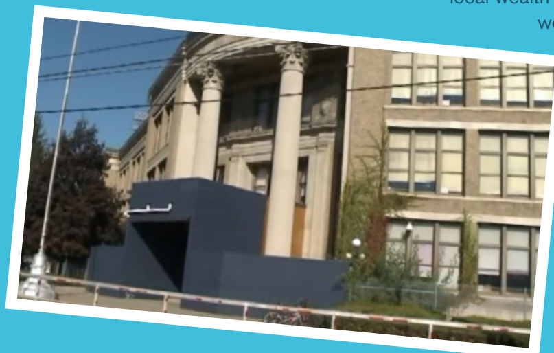
At Meyers High School in Wilkes-Barre, the facade and bricks are crumbling, creating a danger of falling debris. Students and staff enter underneath protective sheds.
